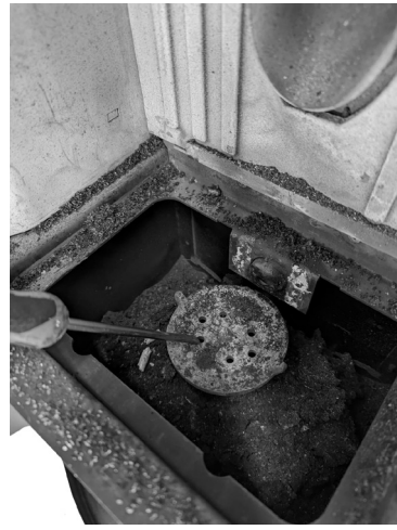
Fig. 37 - Burning pot cleaning
