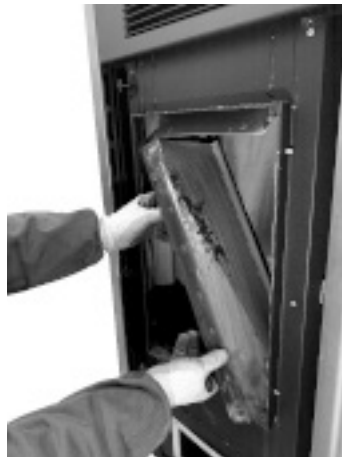
Fig. 50 - Remove the side walls
