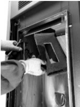
Fig. 49 - Remove the head of the firebox 2
