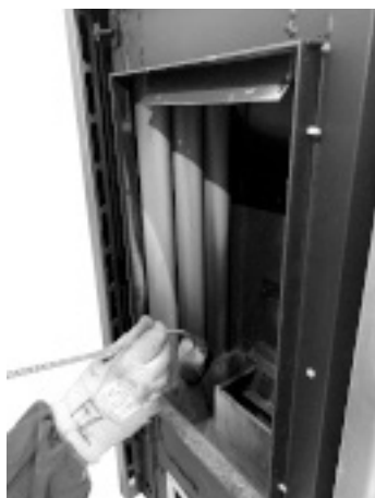
Fig. 52 - Clean with pipe cleaner
