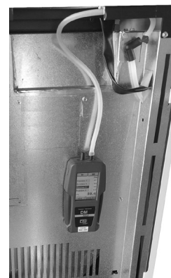
Fig. 37 - Digital pressure switch connection
